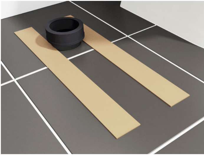
Place the two REGUFOAM® WC-Strips on the floor.
