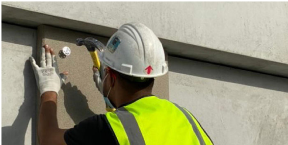
Gently hammer the pin in place
