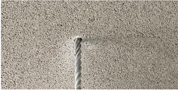
Drill into the centre of the Reapor panel
