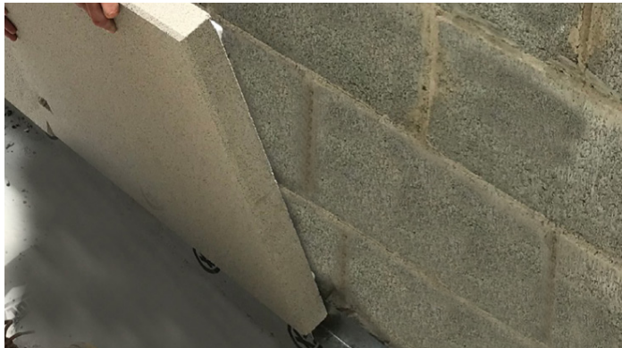
Apply adhesive to the side of the tile only (625 x 208 panels)
