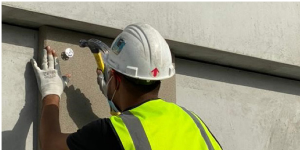
Gently hammer the pin in place
