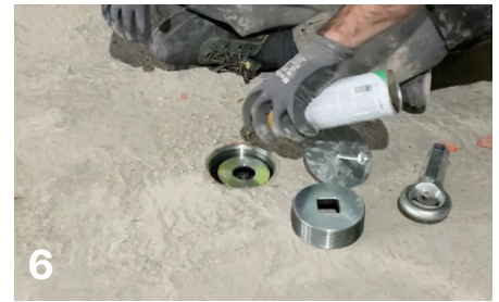
6 Spray lubricant on the top washer
