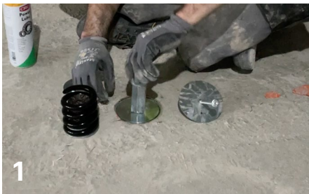
1 Unscrew the lifting washer
