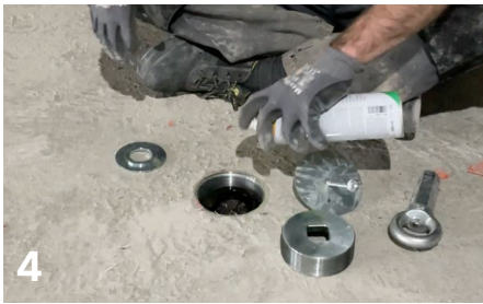
4 Spray lubricant on the top of the spring
