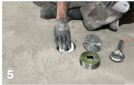
5 Place the top washer on the spring
