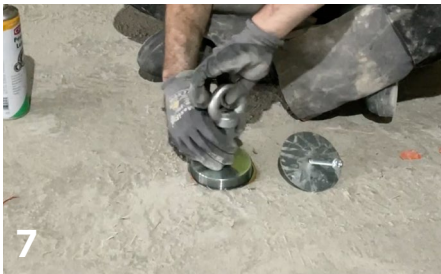
7 Screw the lifting washer back in place
