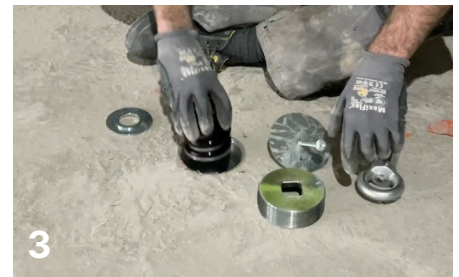
3 Place the spring with the scroll facing down
